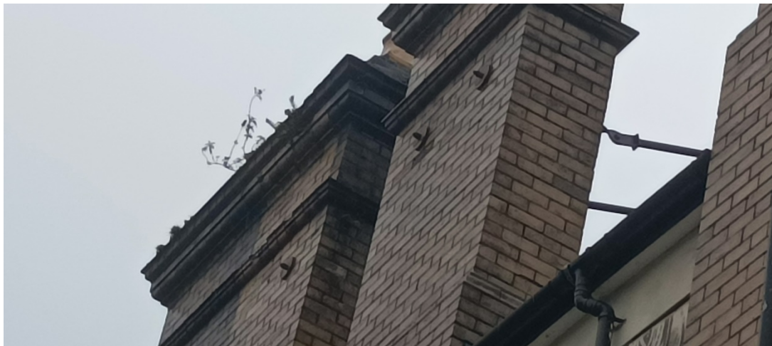
The lack of regular repointing and the failure of the cement render to the rear has permitted considerable water ingress. This will necessitate the removal of all cement render/removal of failed render and its reinstating with a lime render to allow for the drying out of the building's fabric.
